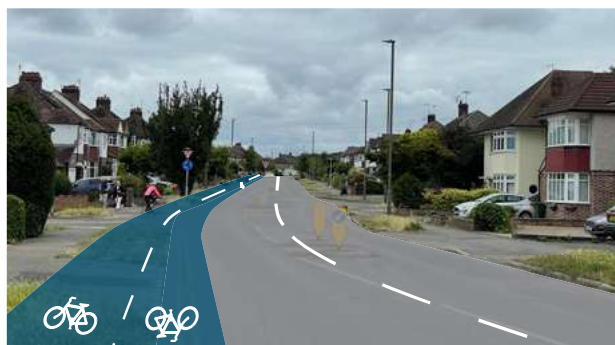
Figure 67. Indicative visualisation of proposed two-way cycle track along Craddocks Ave by reallocating space from the verge and the carriageway.
