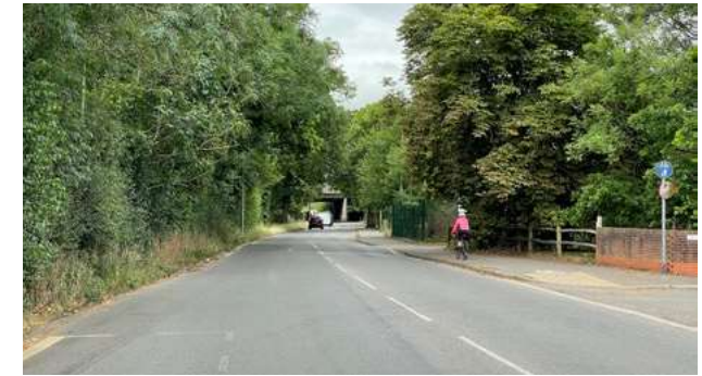
Figure 65. Existing shared use path along Barnett Wood Lane east of the M25 underpass. Available widths can likely accommodate segregation between users.
