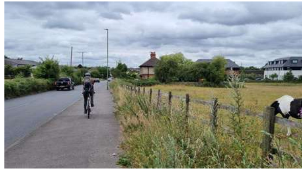
Figure 64. Existing shared use path along Barnett Wood Lane west of the M25 underpass. Existing facility is constrained and segregation likely not feasible within the public highway boundary.
