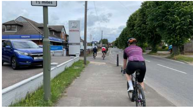
Figure 63. Existing shared use path along Barnett Wood Lane north of Kingston Road to be upgraded to two-way cycle track by reallocating space from the carriageway.
